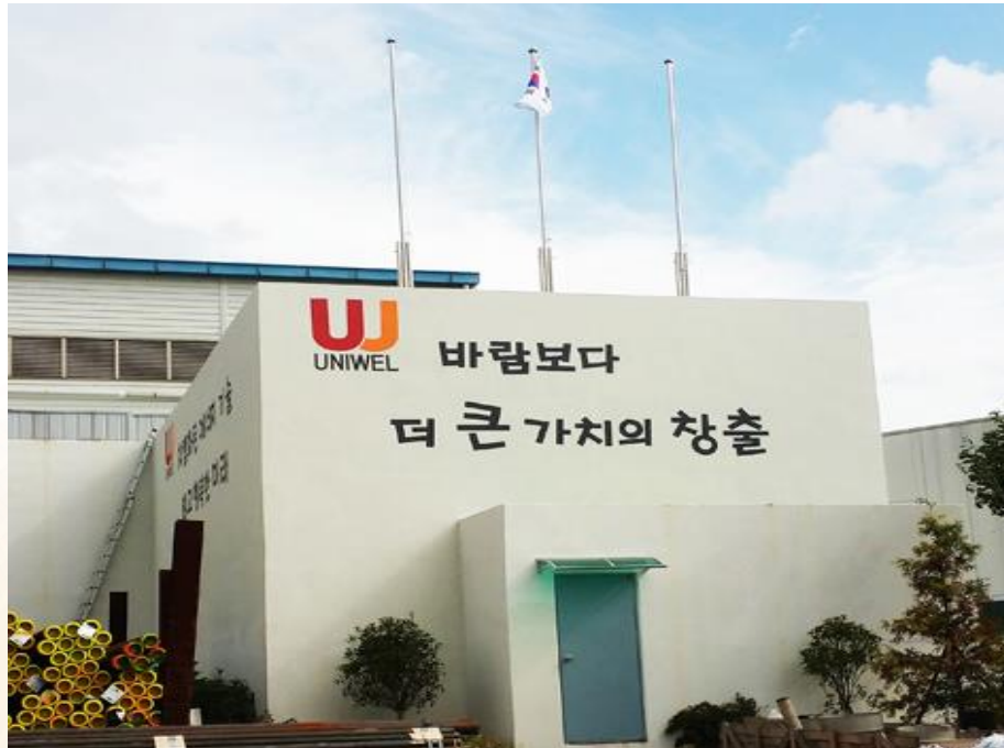
RT Room (in Ulju shop)
